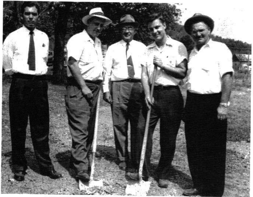
H.E. Harbin Sr., left with shovel and H.E. "Buddy" Harbin Jr., right with shovel, are shown at the ground breaking ceremony for the new Ford dealership to be built on Willow Street in Scottsboro. The ceremony took place, circa 1950.
