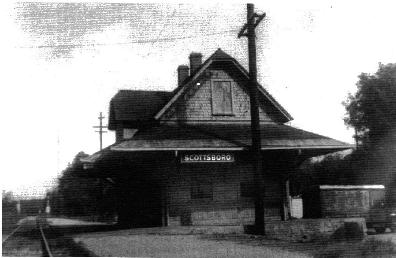
The Scottsboro train depot as it appeared in its heyday. The depot still stands and is in the process of being renovated.
