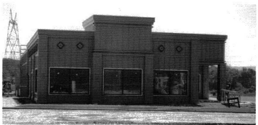
Partially completed Ruby Tuesday Restaurant, located in Scottsboro, September 2000.
